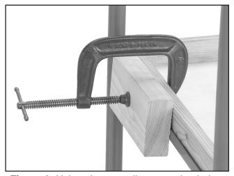
Figure 8. Using clamp to align mounting holes.
